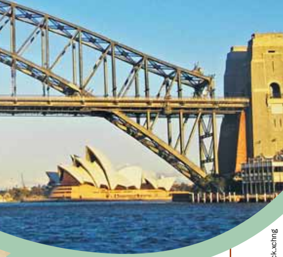
Sydney Harbour Bridge
